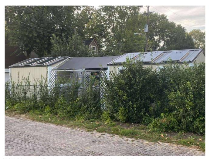
1200 Watts of power installed and tied into an off-grid system housed within the livestock and storage sheds.
