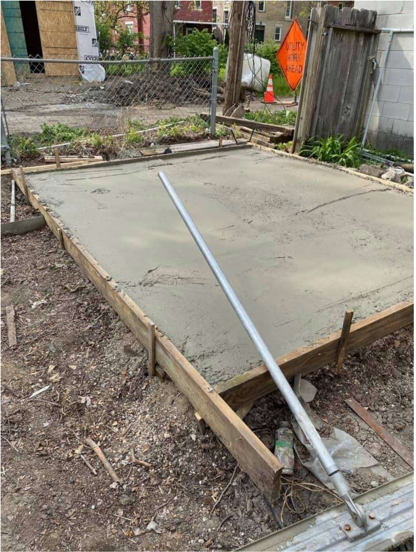
The classroom slab
