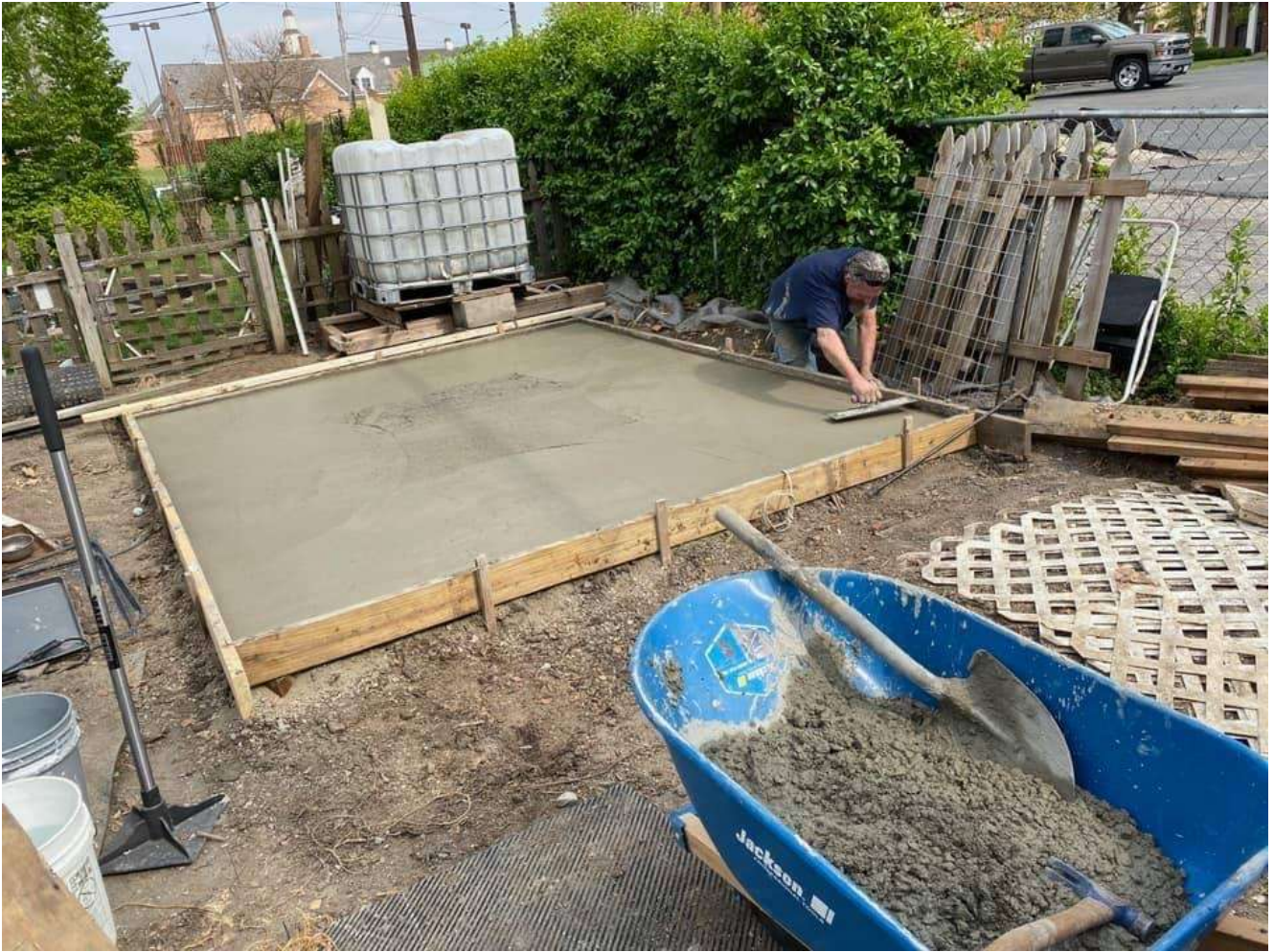
The livestock foundation slab
